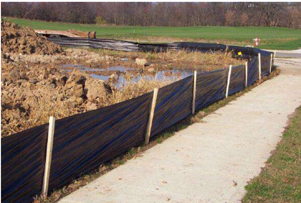
Typical silt fence to be employed
